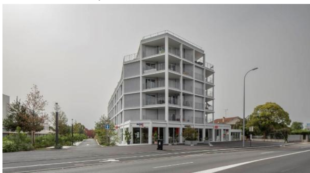
Photo chantier îlot 8.5 – Corylus/P5 (ex CASTORAMA)
