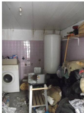
58, rue Lafontaine Expropriation DUP ORI
